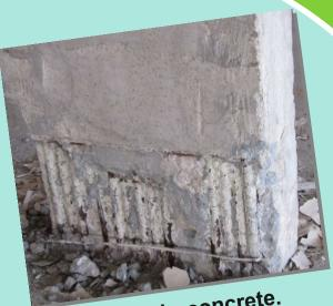
Chlorides & sulphates cause deterioration in concrete.
